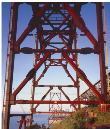
Temporary bridge towers fabricated by AB manufacturing
