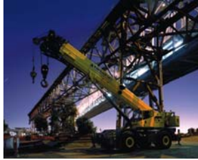
Mating of the OBG in fabricators yard
