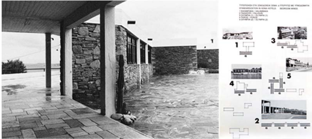
Figures 6,7: Right- Xenia of Mykonos. Architect A. Konstantinidis, left- Standardization in hotels Xenia, wings for rooms, source: Konstantinidis A, 1981. Projects + buildings, A. Konstantinidis, Athens: Agra Ed. and A. Konstantinidis, p.218.
