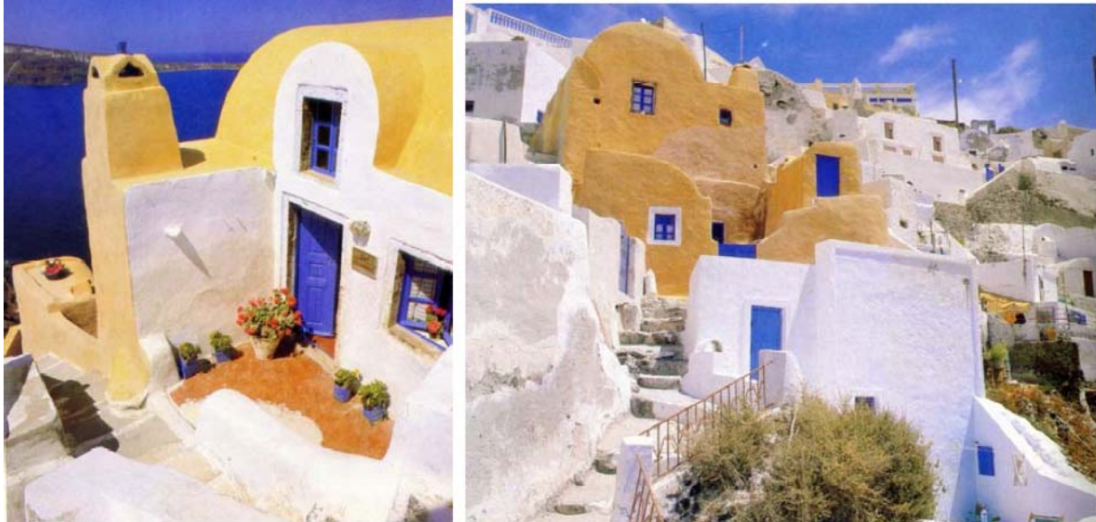
Pictures 1, 2: Oia Santorini, preserved houses through the programme “Preservation and Development of Traditional Settlements in Greece” (1975-1995) GNT0. Source: Collective, (1984). GNT0 Programme 1975-1985 . Athens: GNT0 publications, p. 135 & 146.
