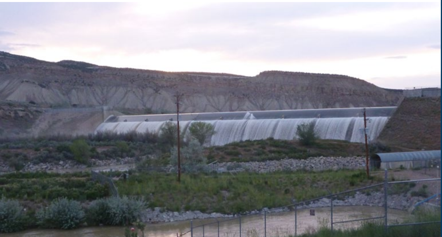
White River spilling over Taylor Draw Dam near Rangely, Colorado
