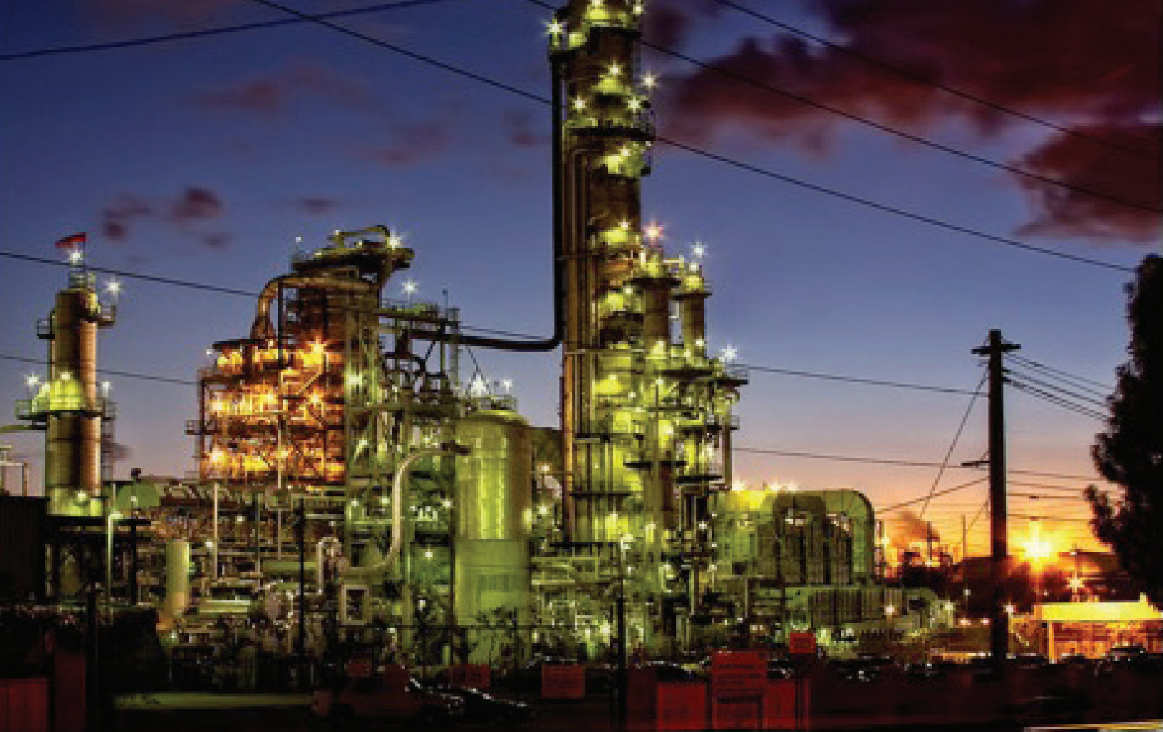
Chevron's El Segundo Refinery, which processes an average of 56,463 barrels of Amazon crude oil every day. While Chevron blames PetroEcuador for its own contamination in the northern Ecuadorian Amazon, its El Segundo refinery is by far the largest non-Ecuadorian refiner of that company's crude. Credit: Pedro Szekeley
