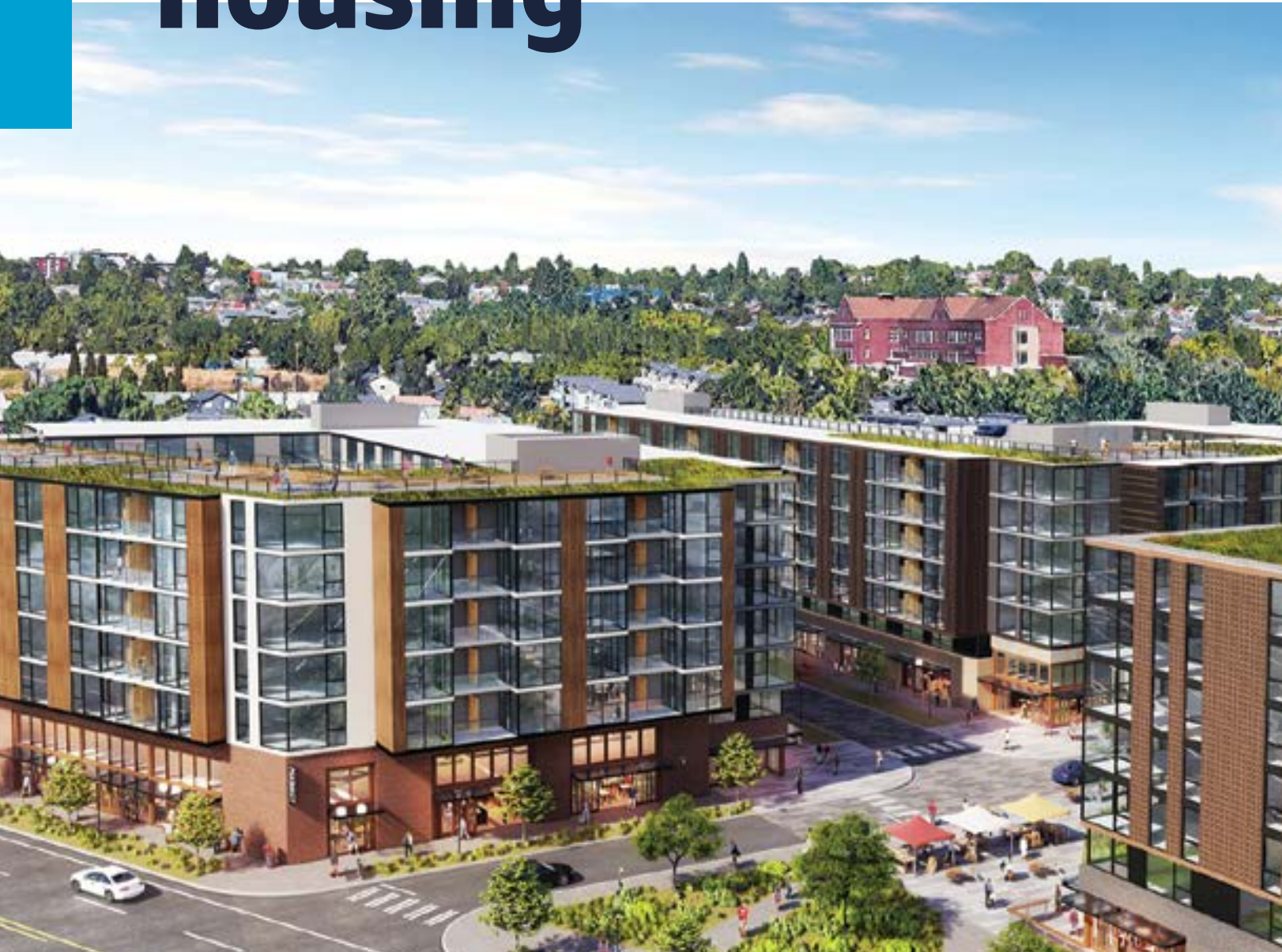
Grand Street Commons, Seattle, WA.
