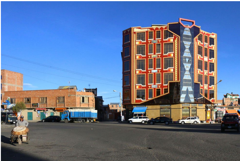
The city of El Alto, a largely informal settlement above the capital La Paz, has changed in the ten years of Evo Morales’s socialist government. Some of the formerly poor have made their mark on the city with palatial new homes called cholets . All photographs by Pedro Rodríguez García.
