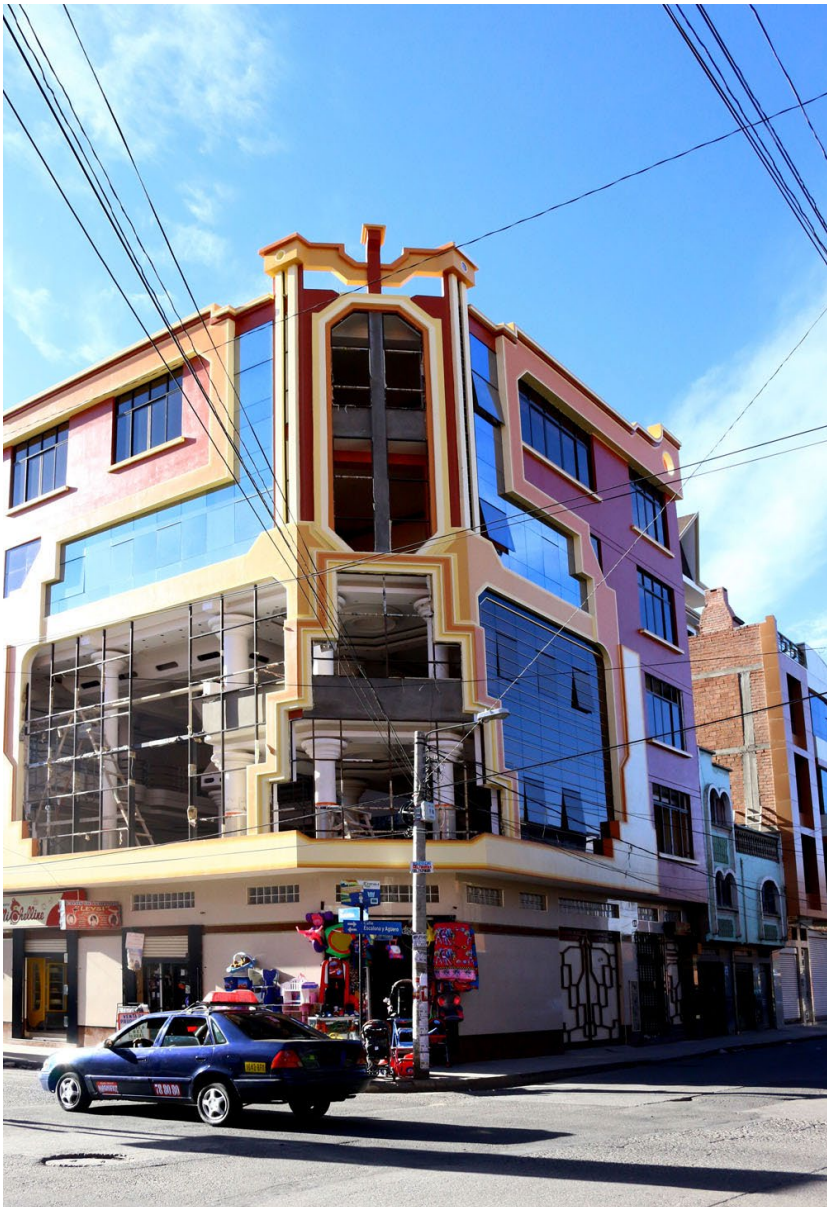
Construction of a cholet in progress.
