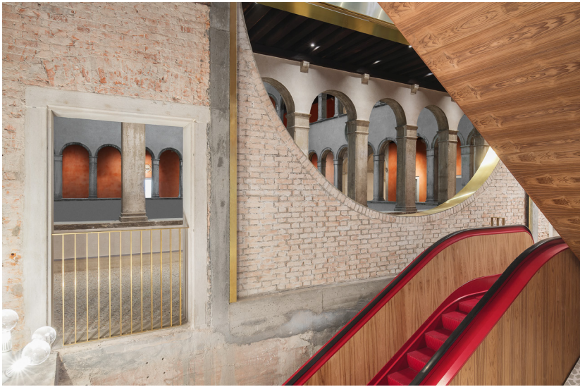
The main escalator crosses a double-height space and is anchored to one of the concrete beams from the 1930s renovation. Photograph by Delfino Sisto Legnani and Marco Cappelletti. Courtesy of OMA.
