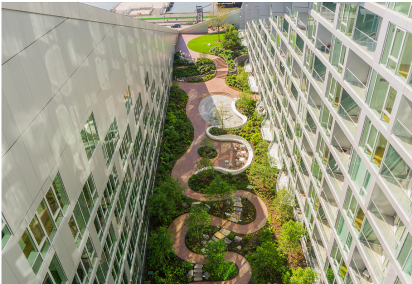
Photograph of interior courtyard, Via 57 West. Courtesy of Starr Whitehouse Landscape Architects and Planners.
