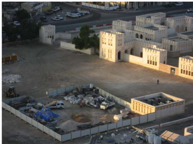
Construction site in Doha, 2013.
