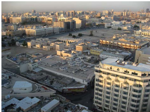
View toward the Msheireb construction site in Doha, 2013.
