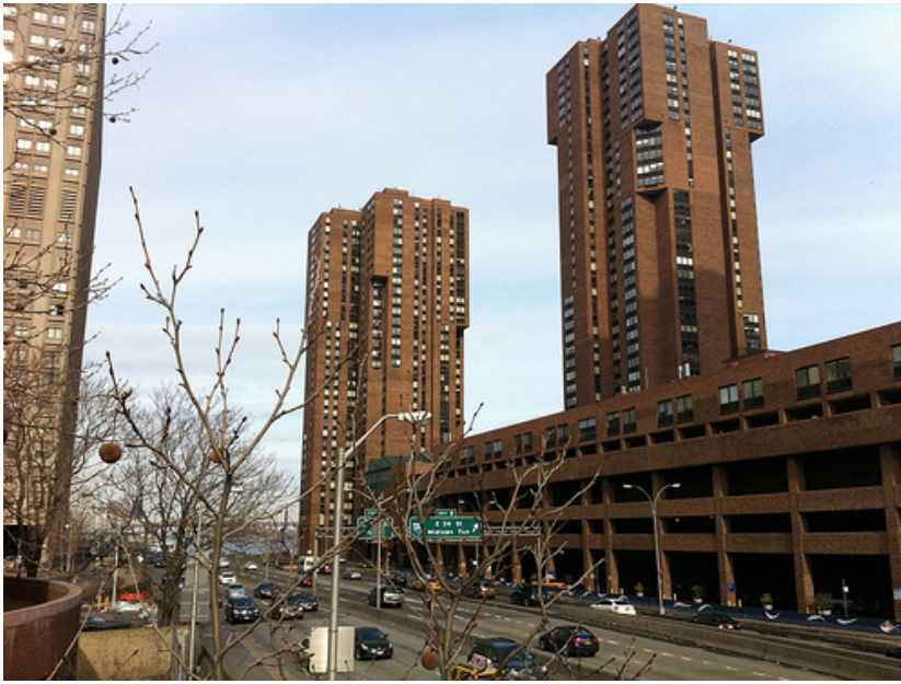
Waterside Plaza looking across FDR Drive at the low bar building, containing parking and entrances at the base and townhouse units at top; photograph taken February 13, 2011. © Teri Tynes.
