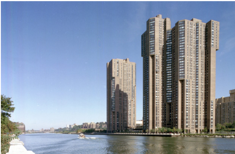
Harlem River Park Towers view from Manhattan shore of the Harlem River looking northeast. Courtesy Davis Brody Bond.
