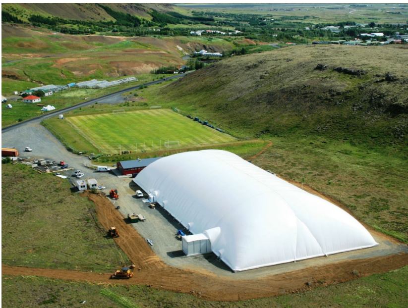
Hamarshöllin, inflated soccer house in Hveragerði, designed by Pro-Ark, 2012. Originally published in “Hamarshöllin,” October 31, 2013, link .
