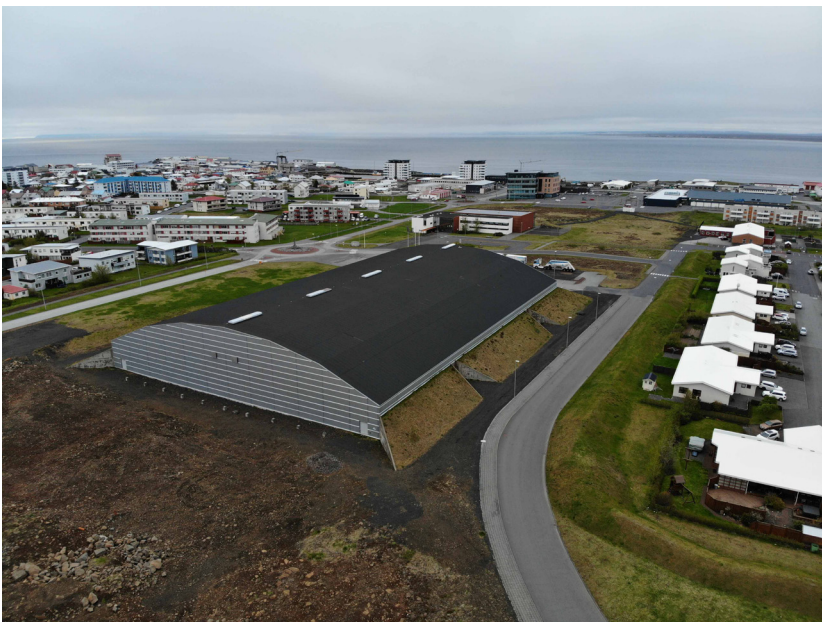
Reykjaneshöllin, Reykjavík, the first soccer house in Iceland, designed by VA Arkitektar, 2000. Photograph by Arnór Sigfússon.
