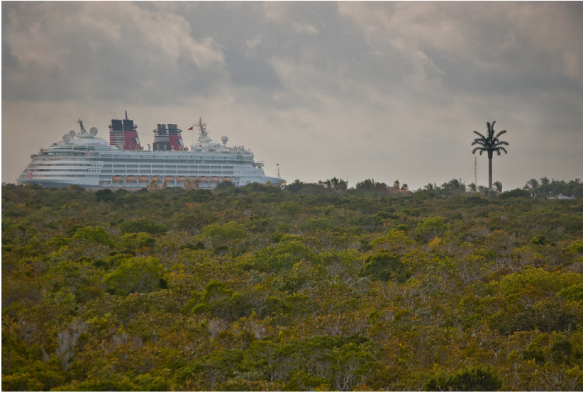
Castaway Cay telecommunications tower disguised as a palm tree. © Scott Sanders.
