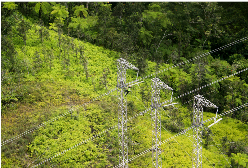
Contractor PowerSecure, Inc., working to restore the electrical grid in the Montaña Area, Caguas, Puerto Rico. Courtesy of the South Atlantic Division, US Army Corps of Engineers.
