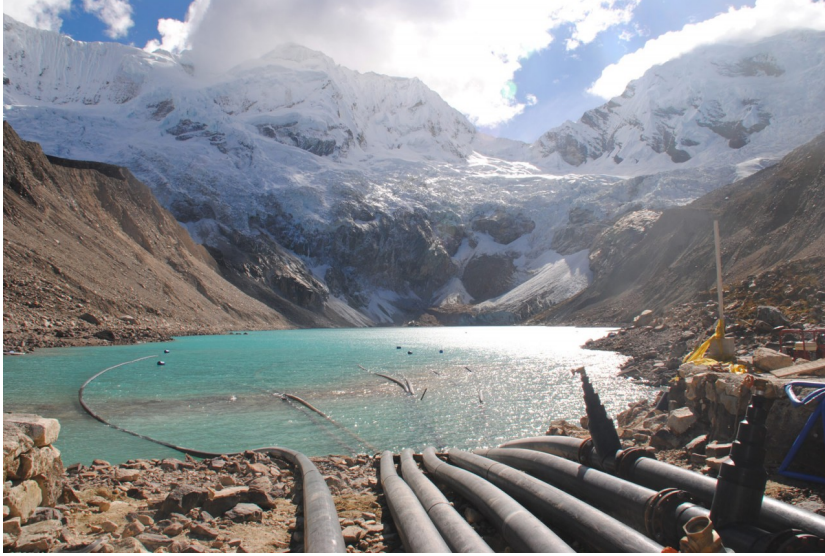
Lake Palcacocha is drained using siphons to avoid Glacier Lake Outburst Floods [GLOF]. Photograph by Mattias Borg Rasmussen.
