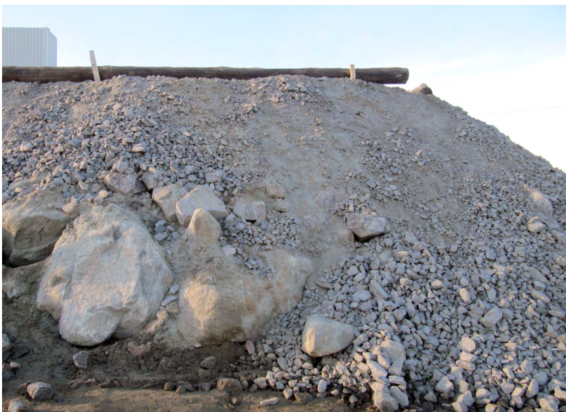
A gravel pad to level the ground by the Clyde River Health Centre. Courtesy of the author.
