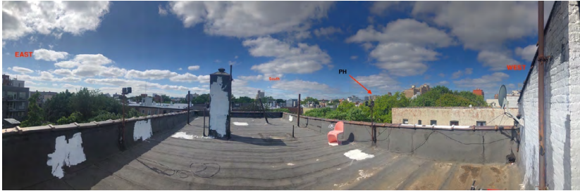
The roof of my old apartment building as pictured by a volunteer NYC Mesh technician. Photo courtesy of NYC Mesh.
