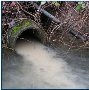
Combined Sewer Overflows (CSOs)
