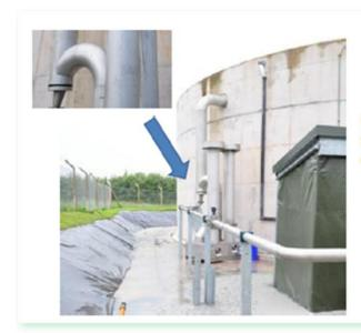
Overflow to PRV very close to reduced size gas pipe. Any foam will quickly enter the PRV
