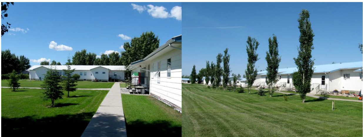
Left: Looking past the kitchen on right to older housing with extensions. Photograph by Simon M. Evans, 2013.
