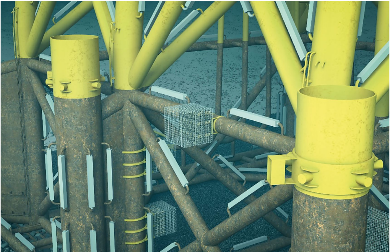
“Fish hotels” on TenneT’s offshore platform in Hollandse Kust Noord wind farm.
