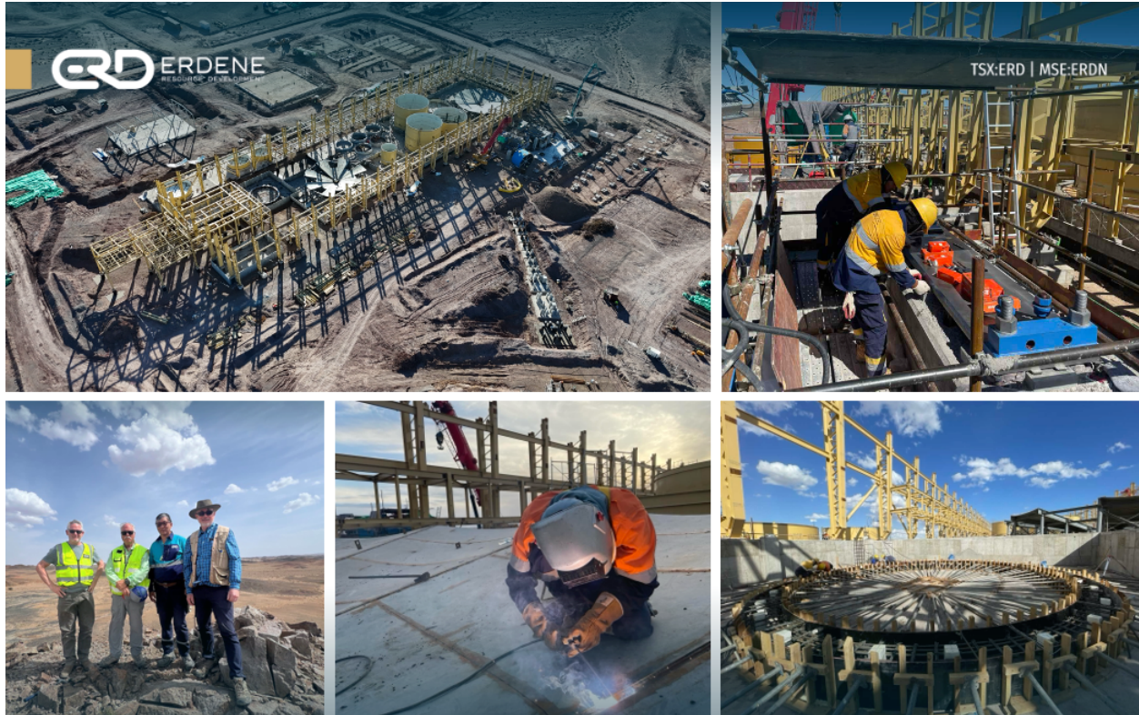
Images: Bayan Khundii Construction Site – August 2024
