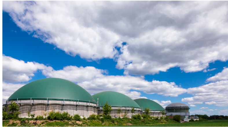
Anaerobic digestors for pig slurry, Germany. Dimitry Naumov.
