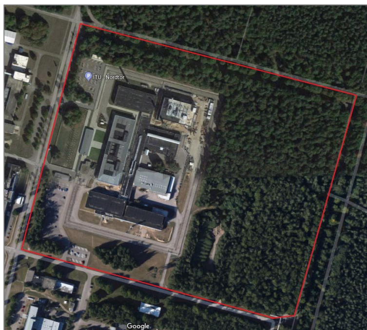
Figure F16: Aerial view of the site including “natural” parts
