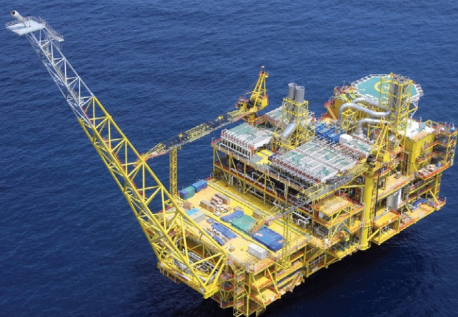
Kebabangan platform, Malaysia
