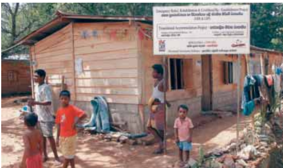
Traditional shelters in Sri Lanka built by Concern.
