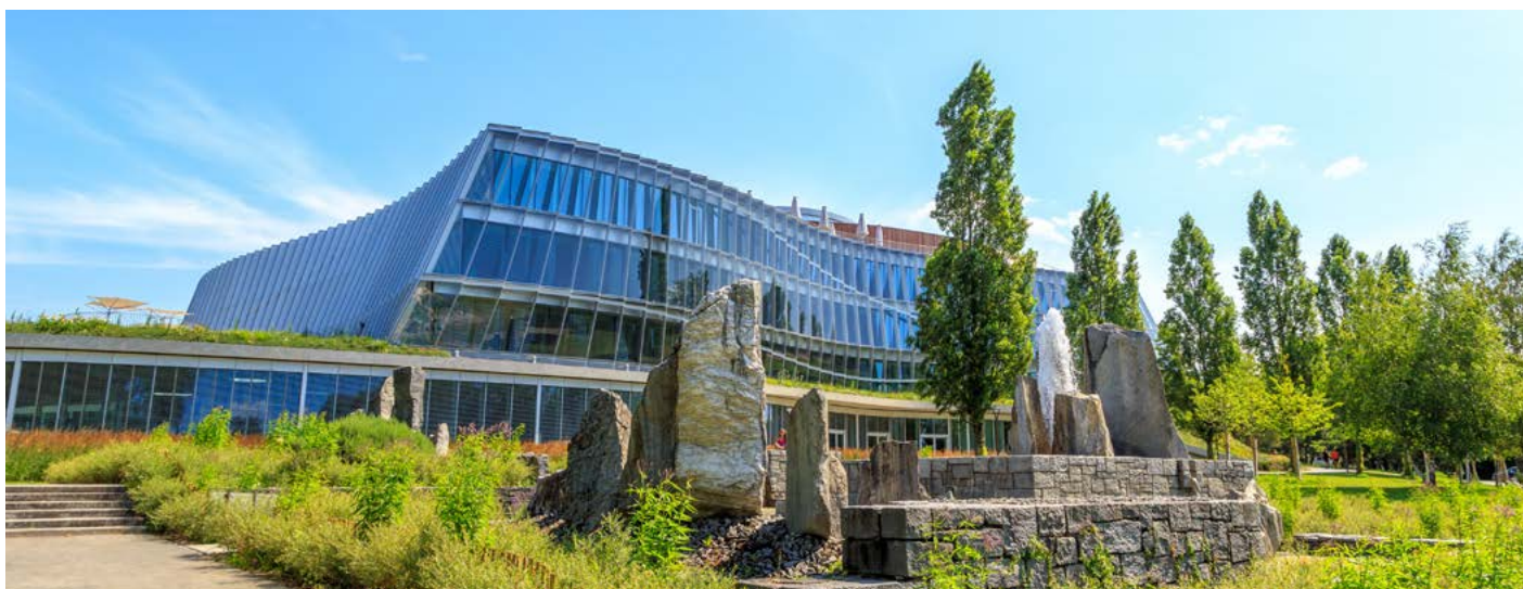
Olympic House has won wide acclaim for its sustainable construction standards. © Maykova Galina
