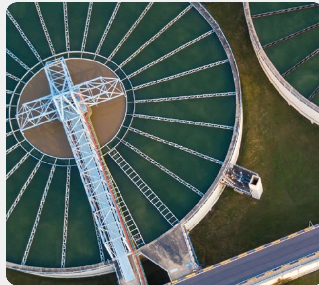
| A wastewater clarification tank used in water recycling.
