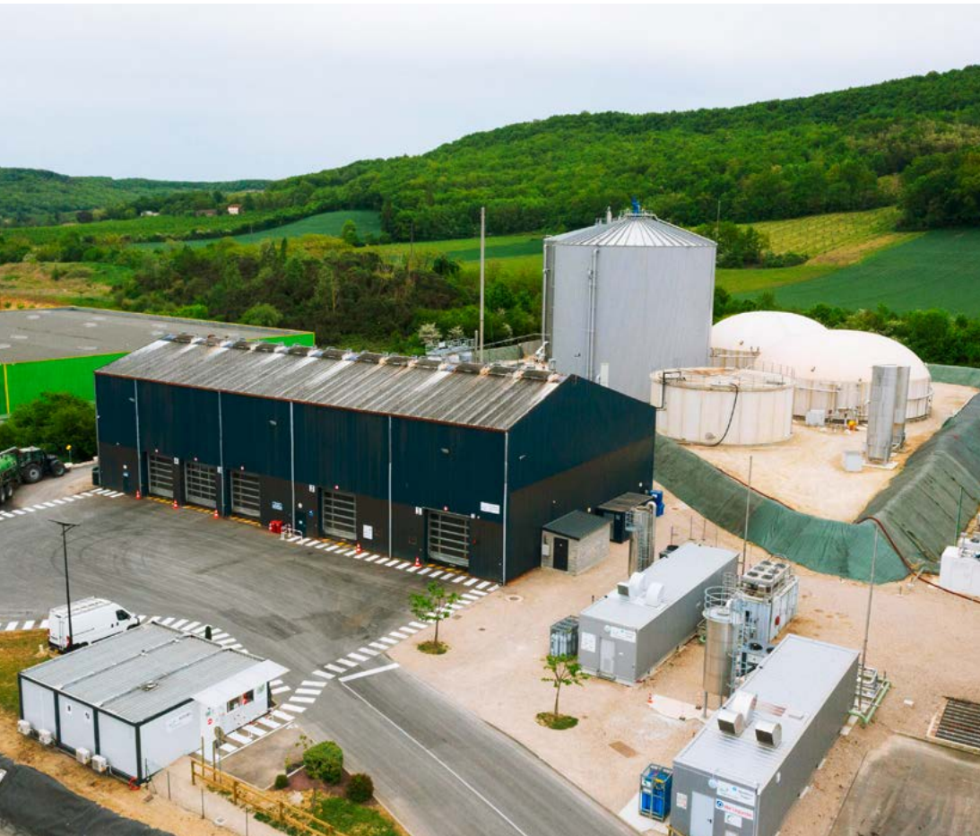
The BioVilleneuveois methanization plant in Villeneuve-Sur-Lot (France).
