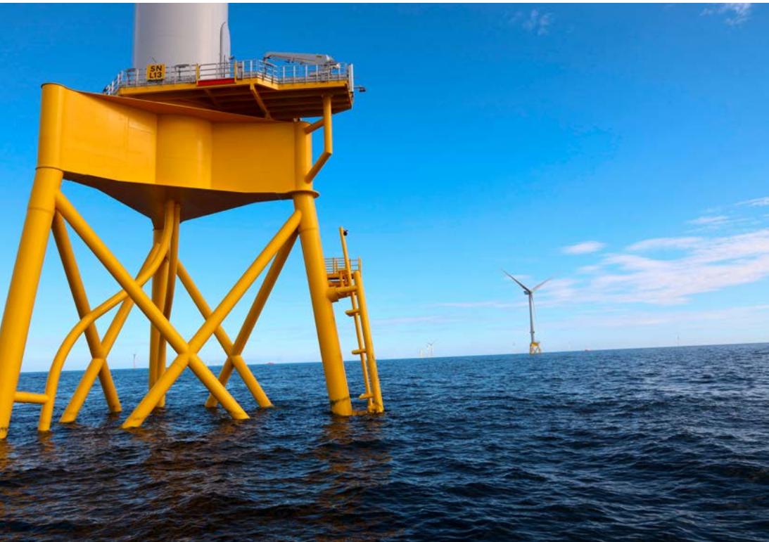
Seagreen (Scotland) offshore wind farm under construction.
