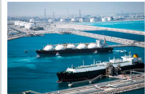
Ras Laffan liquefaction terminal, Doha (Qatar).
