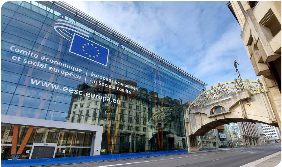
© Architecture: Art & Build + Atelier d'architecture Paul Noël
