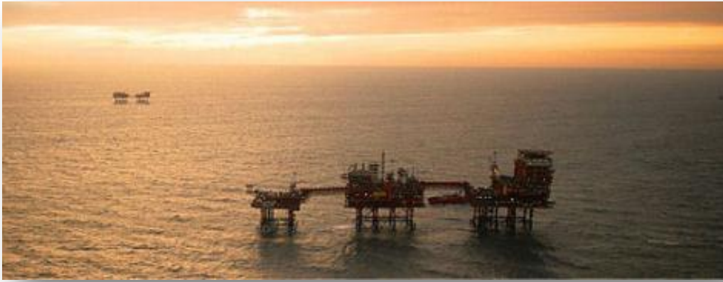
Gas and CO 2 Storage
