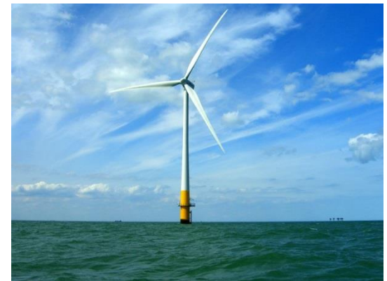
Offshore Wind energy
