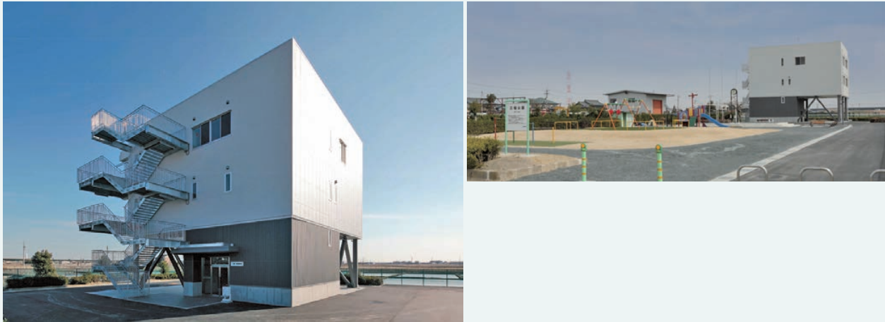
Tsunami evacuation tower built by Tobishima Village, Aichi Prefecture. Source: OYO Corporation.
