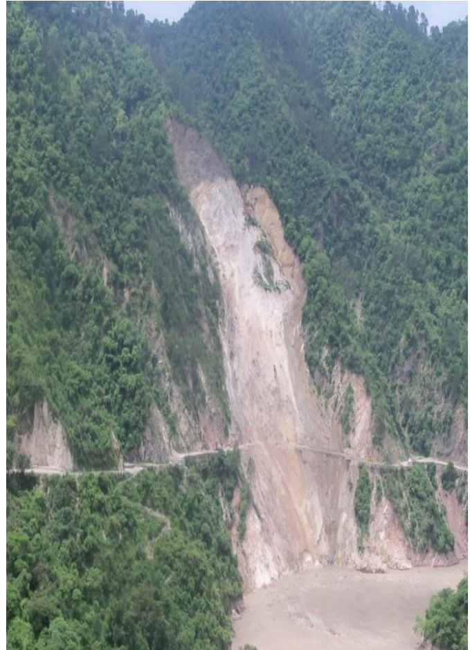
View of Kaliasaur Landslide in 2013
