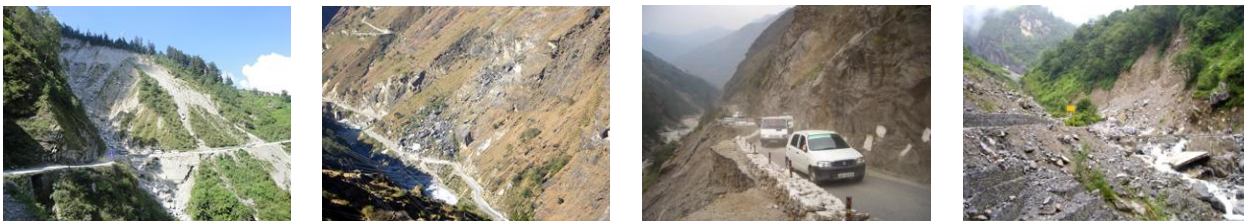
A few problematic landslides along Chamoli-Badrinath sector of NH-58
