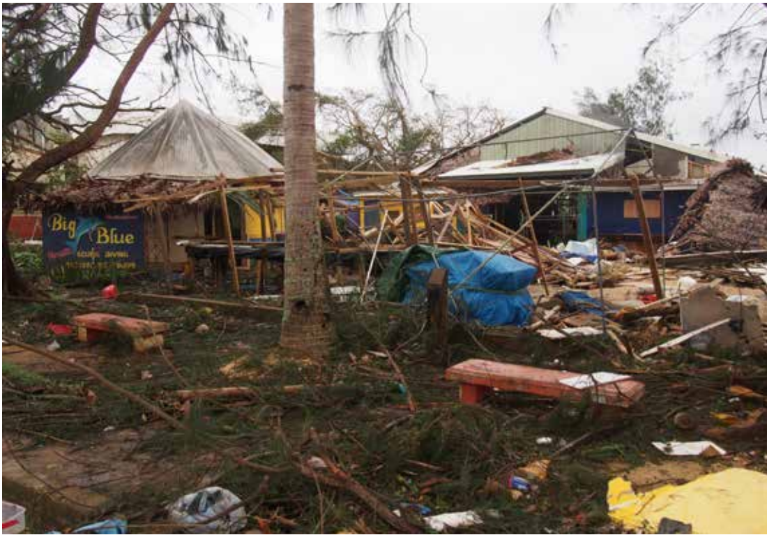
Damage to Port Vila foreshore, including many tourism businesses. © Becky Last, Vanuatu Dept. of Tourism.
