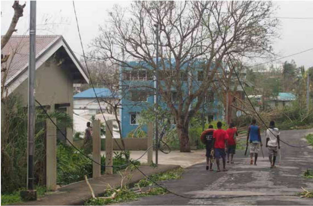
Men walk by damaged power lines in Port Vila. © Becky Last, Vanuatu Dept. of Tourism.
