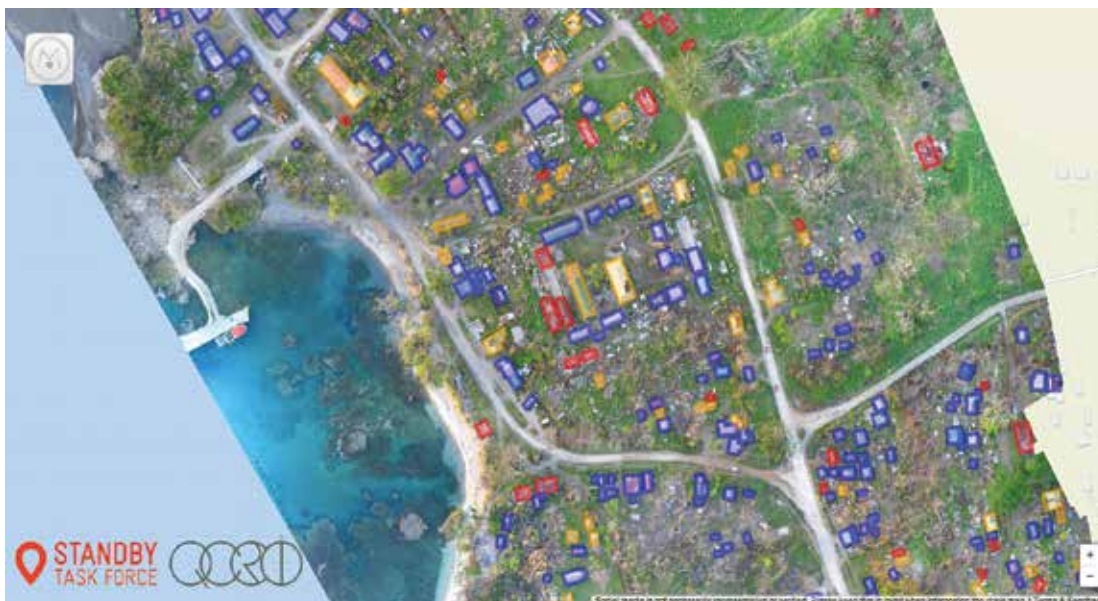
Damage to buildings mapped from X-craft footage. Source: Micromappers.
