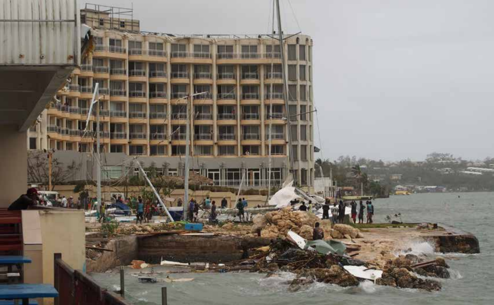
Damage to Port Vila waterfront. © Becky Last, Vanuatu Dept. of Tourism.
