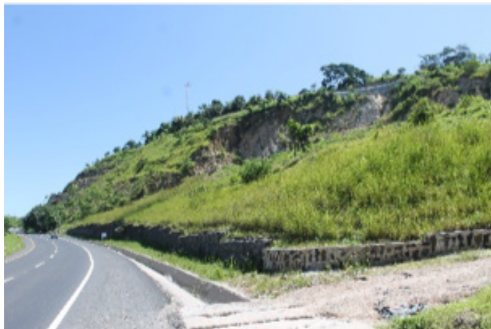
Photo 4.1: Vegetation at a Road Mountainside Slope
