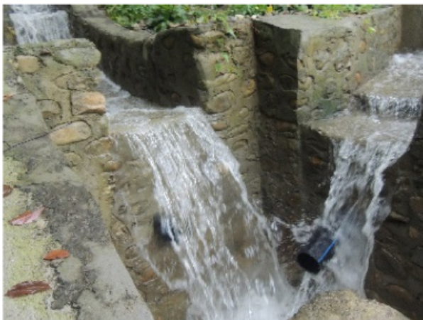
Photo 4.2: Surface-Groundwater Collecting Conduit with Ground Surface Drainage at Catch Pit
