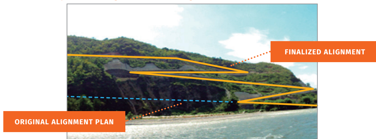
Photo 3.2: Example of Road Alignment Plan Avoiding Geohazards
