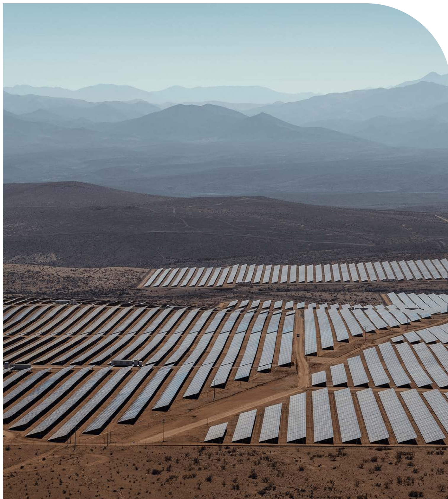
El Romero solar farm in Chile (80 MW for Google)
