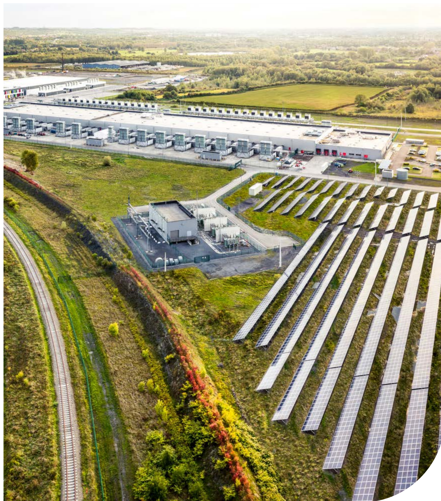
Google's data center in St. Ghislain, Belgium.
