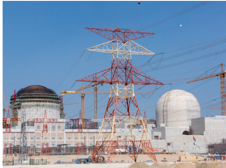
Construction works at the Barakah nuclear power plant, United Arab Emirates.
