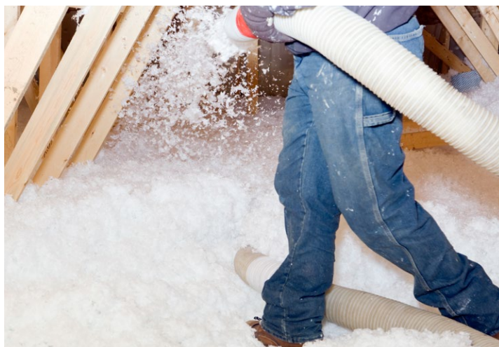
Scaling up insulation (pictured) and other buildings energy efficiency improvements are foundational to keeping energy affordable and achieving our net zero future.
