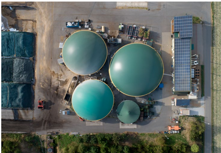
RNG facilities (pictured) capture methane from waste – preventing emissions into the atmosphere – and create a valuable product to use in heating.
