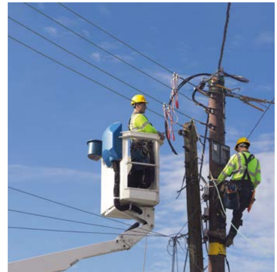
→ Work at height and electrical work related to roll out of networks requires us to insist on strict health & safety requirements for all those working on behalf of Nokia.
