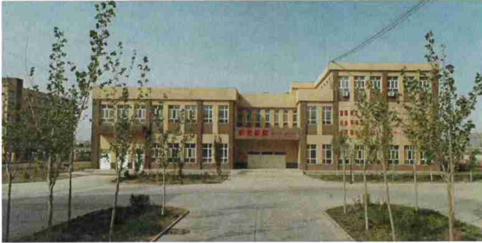
Teaching building of a vocational education and training center in Kashgar City of Xinjiang
