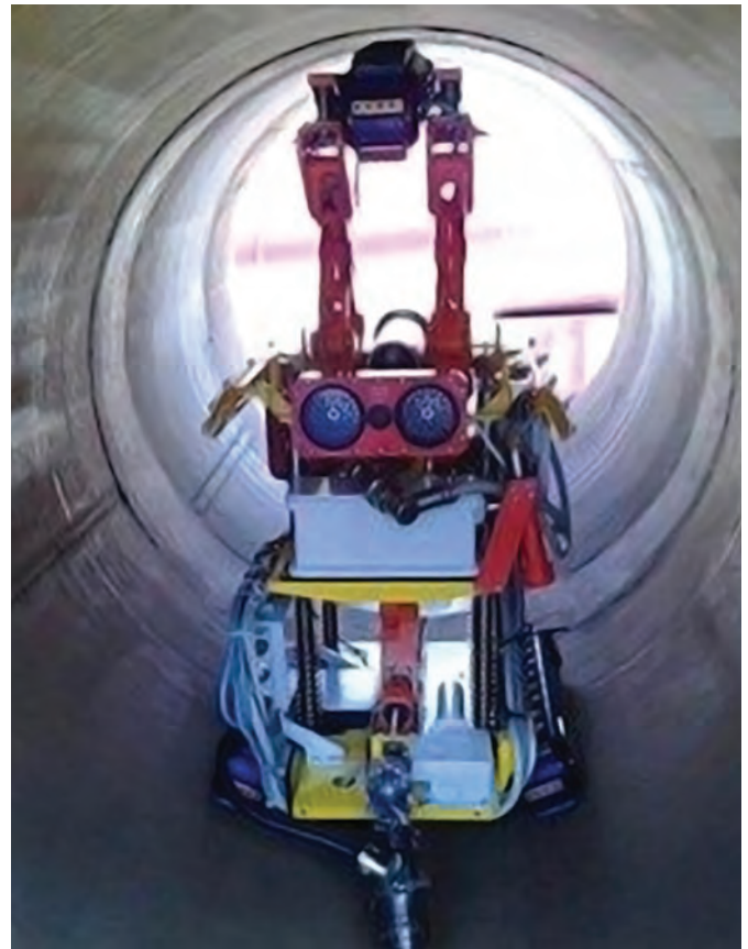
Robotic crawlers such as this one are now used to examine the interior of the pipes.
