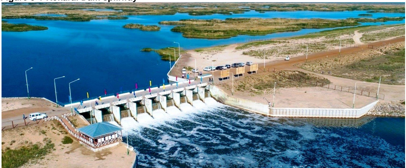
Figure 3-1 Kokaral Dam spillway
